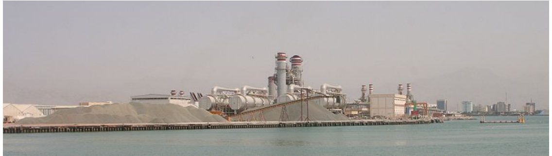
Figure 3: Water desalination plant in Ras Al Khaimah, United Arab Emirates. Attribution: Wikimedia Commons
